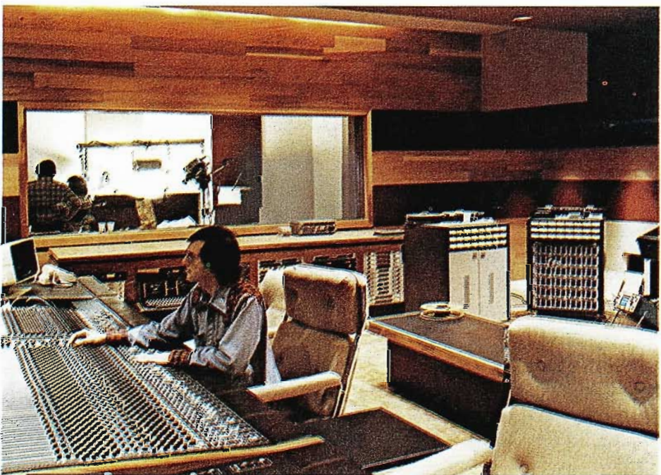
Sophisticated Audio Sweetening Room includes a custom computerized-controlled audio console. A window in the background provides a view of the soundstage.
