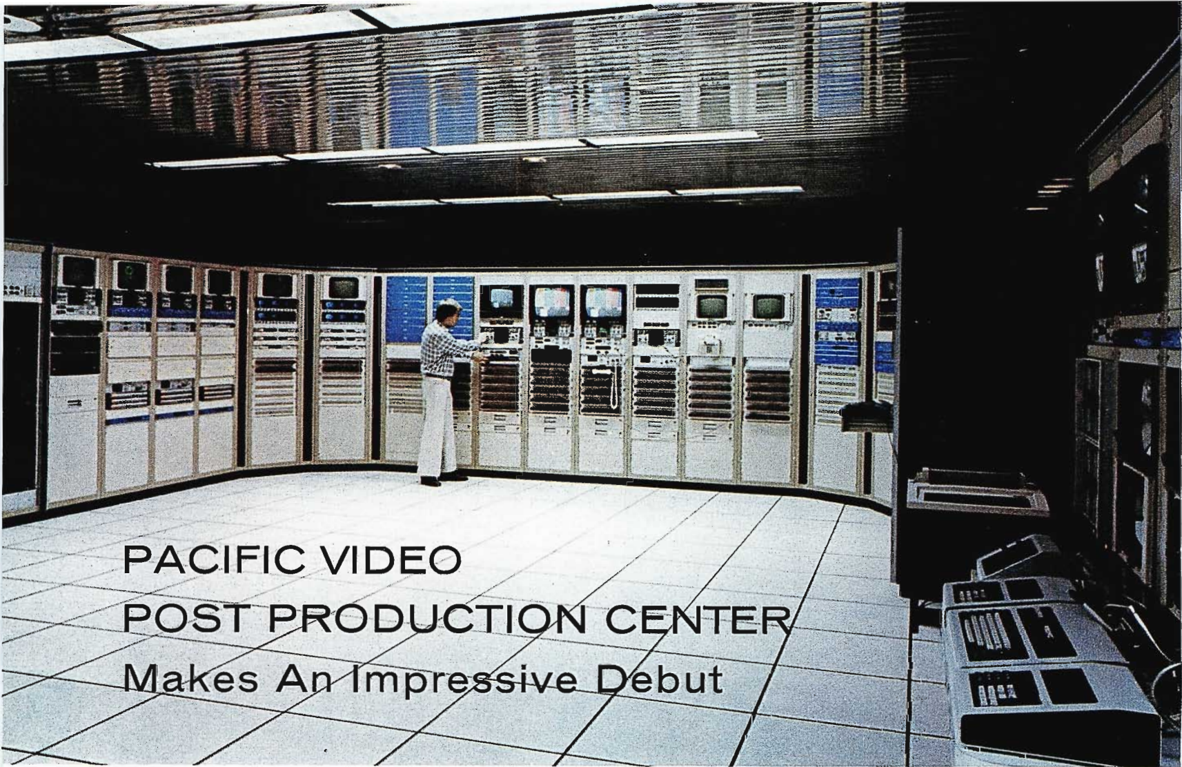
Master Control is an exotic, functional area which provides centralized system control and full accessibility to the equipment components.
